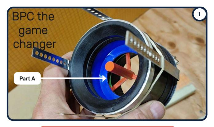
**Do not remove the red "Blocking Spider" (part A)** until ready to engage the BPC with the drain outlet!
