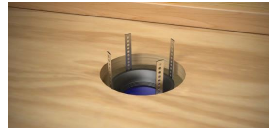
BPC ALWAYS INSTALLS TO SAME DEPTH
