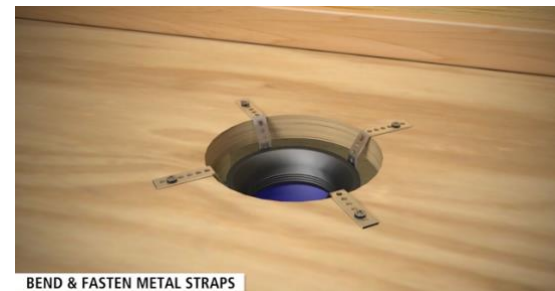
BEND & FASTEN METAL STRAPS
